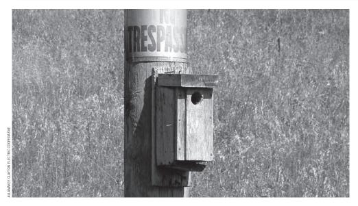
A sign and bird house are illegally attachment to an electric pole. These items and their sharp nails or staples can injure line technicians or puncture their protective gloves.
